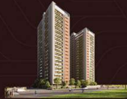
Iscon Ambli Road PR/GJ/AHMEDABAD/AHMEDABAD CITY /AUDA/RAA09547/251221
